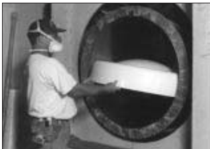
End section is inserted into position determined by desired capacity.
